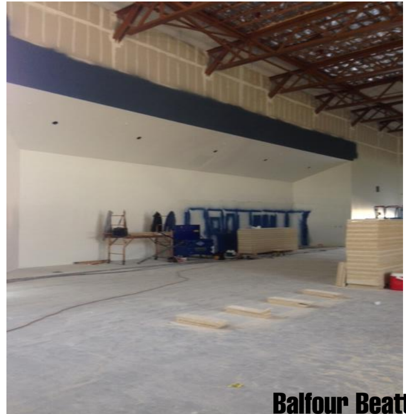
PAINTING HAS STARTED AT THE VISITOR'S SIDE OF THE GYM
