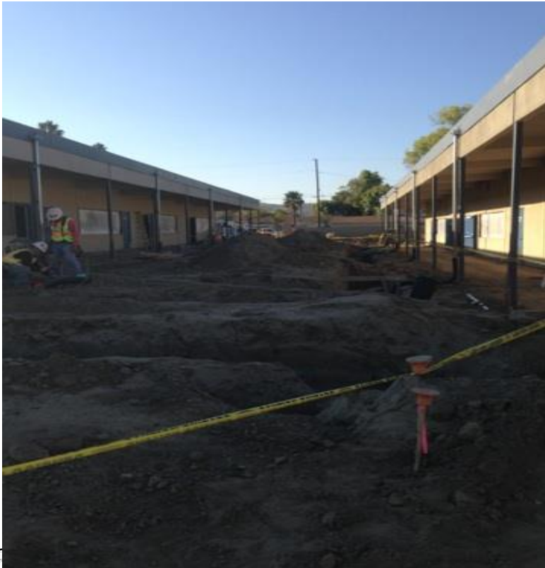
DIGGING FOR FOOTING FOR PLANTERS, STAIRS AND WALKWAYS 10/16/2013
