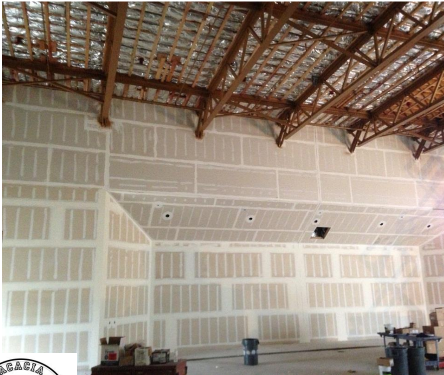
DRYWALL FINISHES ARE COMPLETE
